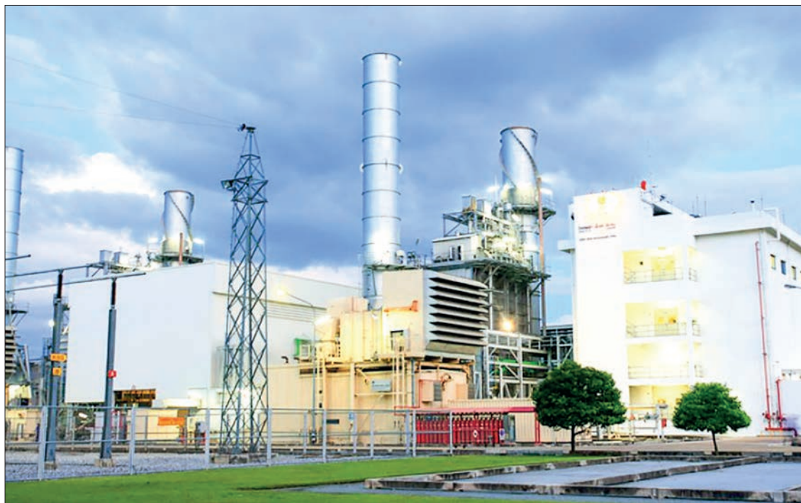
The picture shows the power sub-station being constructed with foreign direct investment.
