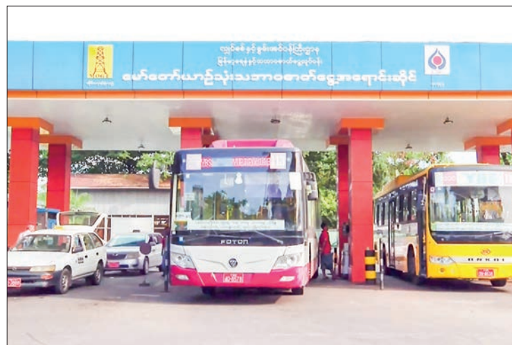
One of the natural gas fuel stations in Yangon.
