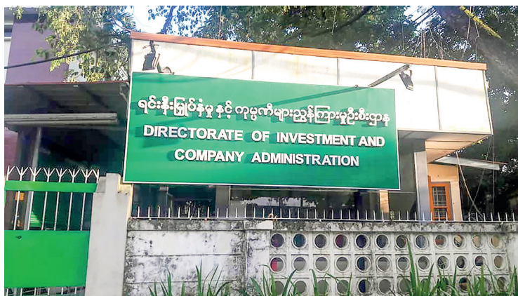
The photo shows an office building of Directorate of Investment and Company Administration-DICA.
