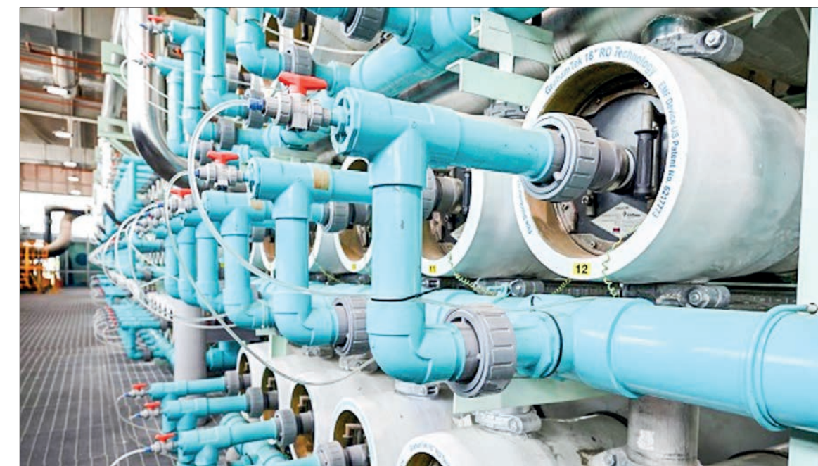
This picture taken on 27 July 2021 shows the reverse osmosis treatment on used water equipment at the Bedok NEWater plant in Singapore. Giant pumps whirl deep underground at the plant in Singapore that helps transform sewage into water so clean it is fit for human consumption while reducing ocean pollution. PHOTO: REPRESENTATIVE IMAGE/ ROSLAN RAHMAN / AFP
