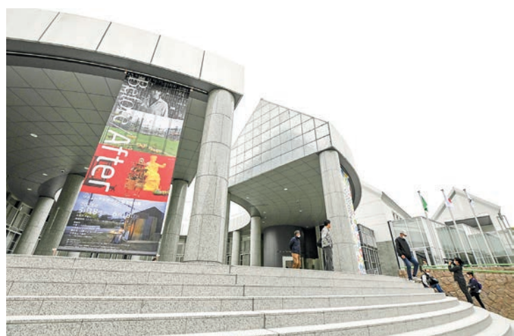
Photo shows the exterior of the renovated Hiroshima City Museum of Contemporary Art on 17 March 2023. PHOTO: KYODO
