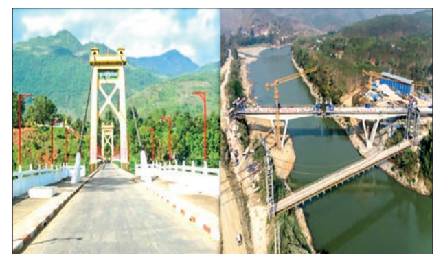
The general view of the new construction of the Kunlong Bridge.
