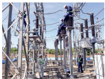
Regular maintenance work is being done at the 230 KV substation.
