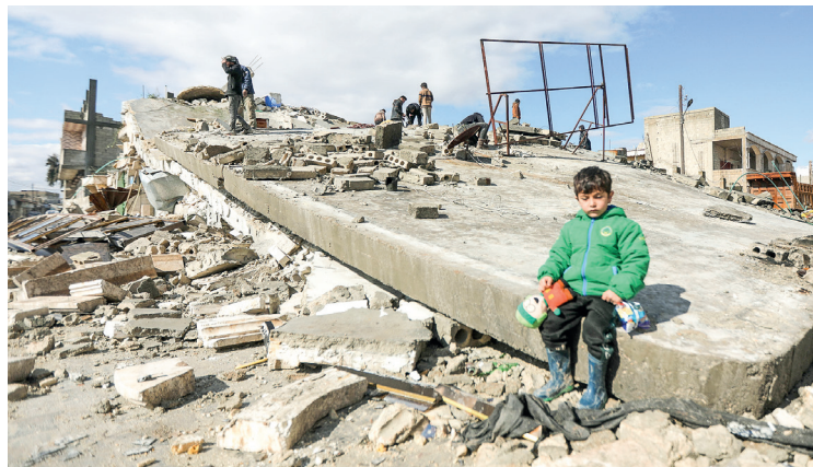
A Syrian child sits on a collapsed building in the town of Azaz on the border with Türkiye on 7 February 2023, following a deadly earthquake. The Syrian Red Crescent appealed to Western countries to lift sanctions and provide aid after a powerful earthquake has killed more than 1,600 people across the war-torn country. PHOTO: AFP
