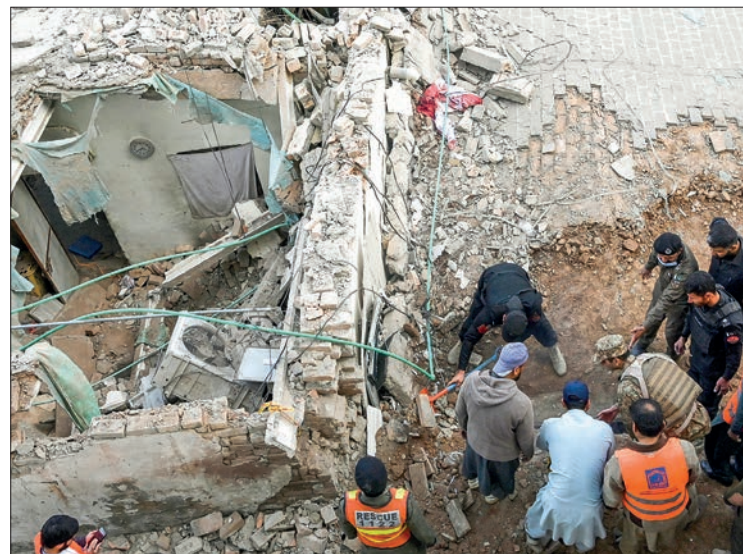
Security personnel and rescue workers prepare to search for the blast victims in the debris of a damaged mosque inside the police headquarters in Peshawar on 30 January 2023. PHOTO: AFP
