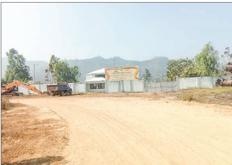
The photo shows a section of the Paletwa-Zorampur road under implementation.
