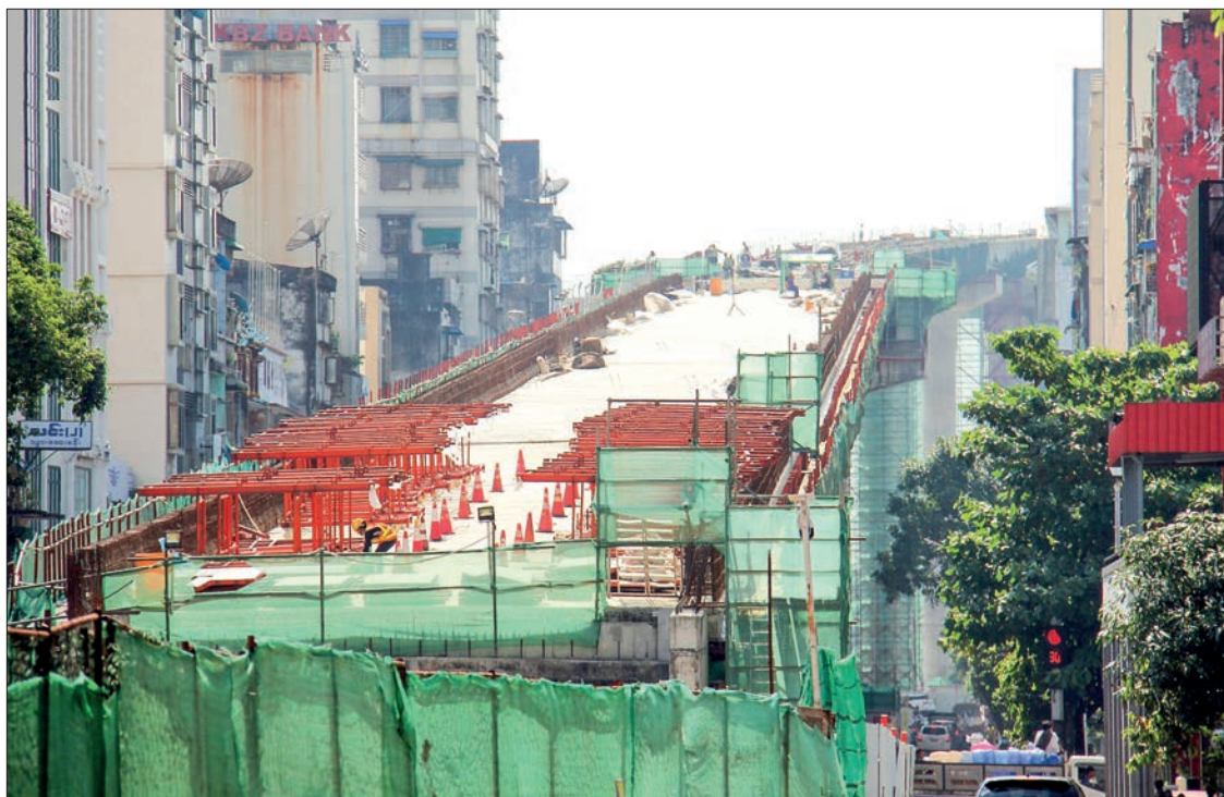
The photo shows a partial completion of the bridge construction.
