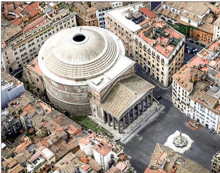
The Pantheon in Rome features the world's largest unreinforced concrete dome. PHOTO: AFP
