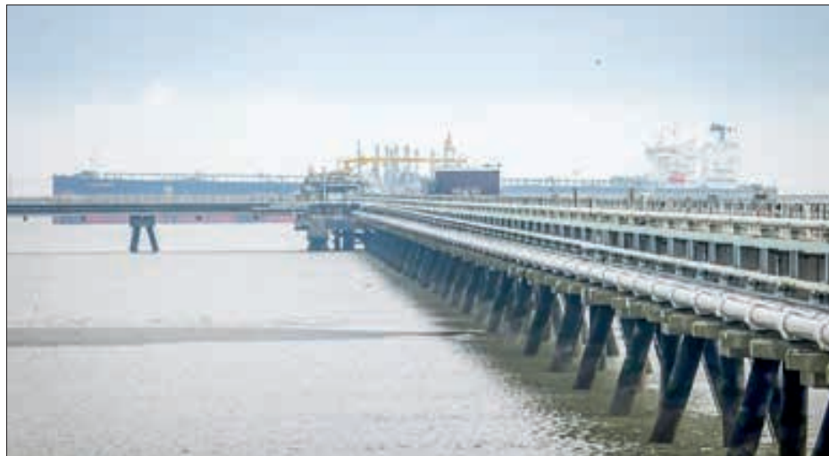
LNG terminals allow for the import by sea of natural gas chilled to liquid form to facilitate transport. PHOTO: AFP/FILE
