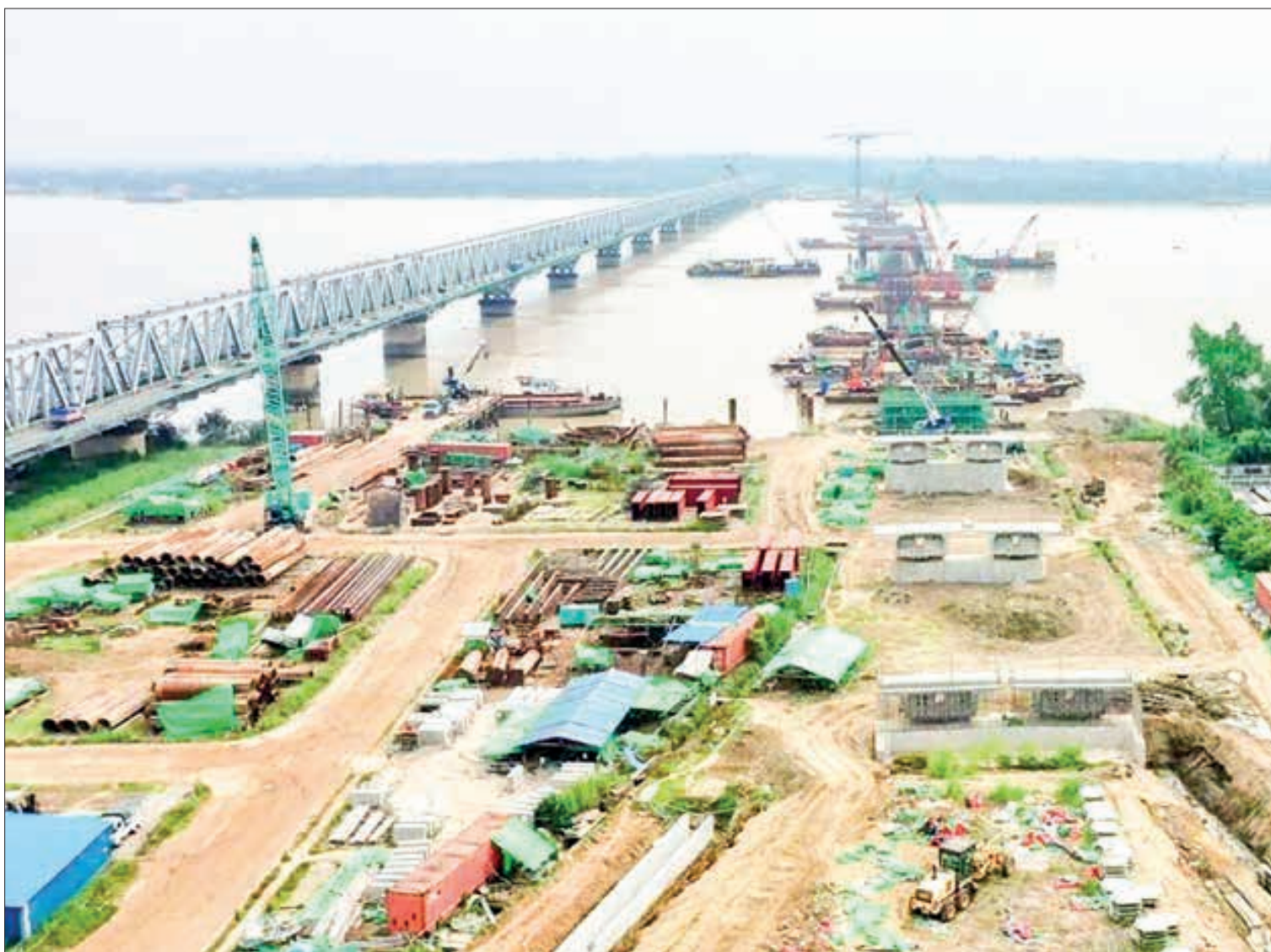
Part 2 construction site of bridge. PHOTO: SOE MYINT AUNG
