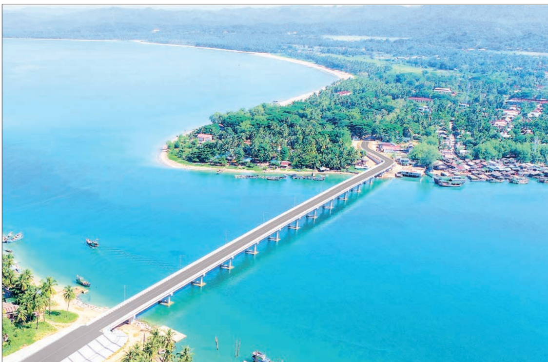
An aerial view of the Gwa Chaung Bridge.
