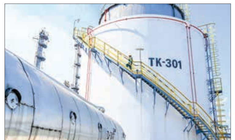
A worker takes the stairs outside a giant tank at the Duna (Danube) Refinery of Hungarian MOL Company located near the town of Szazhalombatta, about 30 kilometres south of Budapest on 5 May 2022. PHOTO: ATTILA KISBENEDEK / AFP
