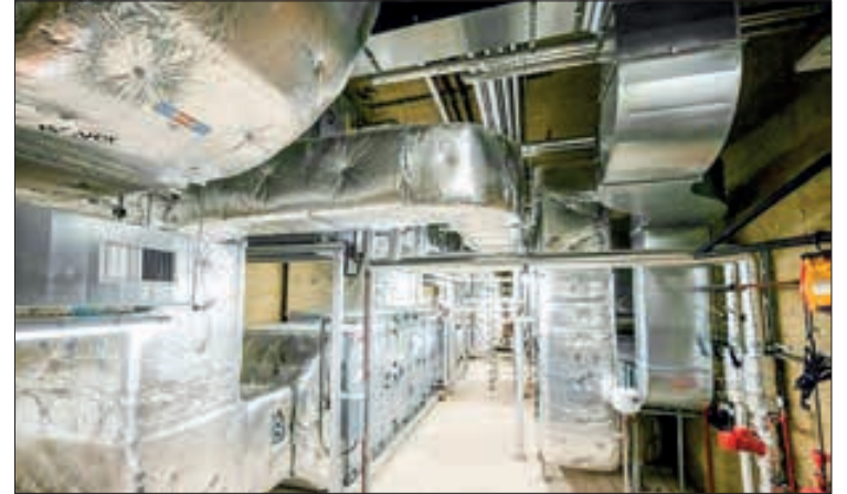
This energy-efficient system sucks warm air from outside to heat air/water inside the building. PHOTO: AFP
