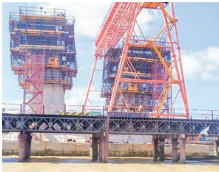
Some parts of the construction of the Yangon-Dala River Bridge.
