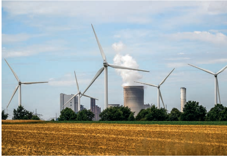
Wind turbine are seen in front of a coal-fired power plant operated by German energy supplier RWE in Niederaussem, western Germany, on 13 July 2022. PHOTO: AFP
