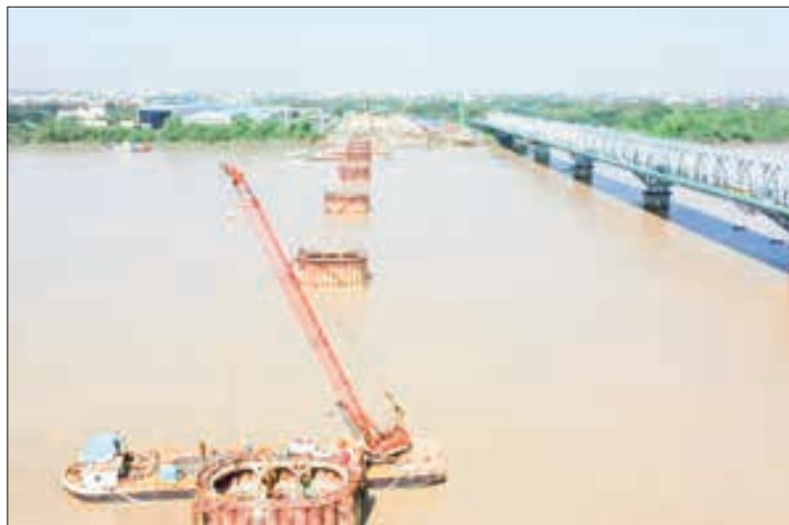
A new Thanlyin Bridge is under construction.
