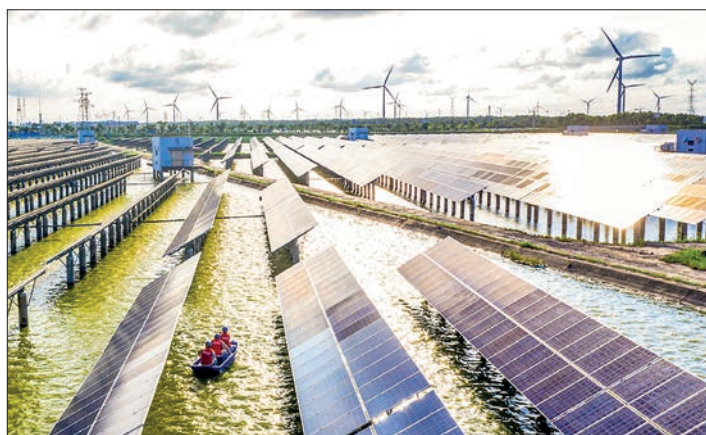
Electrical workers check solar panels at a photovoltaic power station built in a fishpond in Haian in China's eastern Jiangsu province. PHOTO: REPRESENTATIVE IMAGE/AFP
