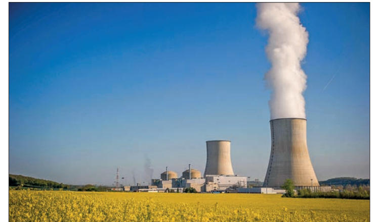
The Civaux nuclear power plant. PHOTO: GUILLAUME SOUVANT / AFP
