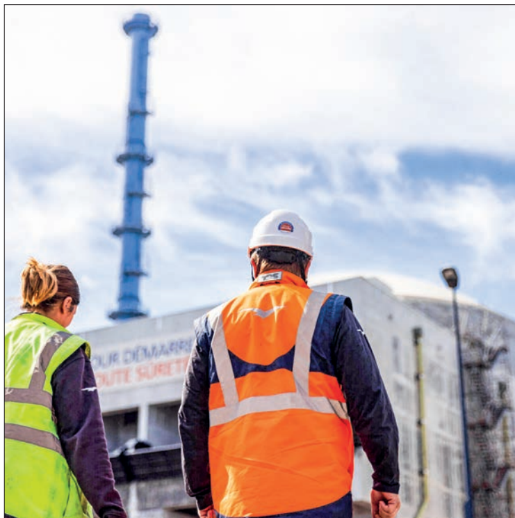
Workers walk past a reactor building at the third-generation European Pressurized Reactor project (EPR) nuclear reactor in Flamanville, Normandy, France on 14 June 2022. PHOTO: SAMEER AL-DOUMY /AFP
