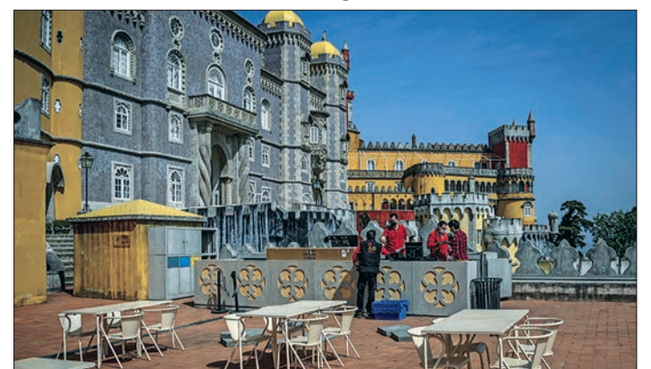
Technicians work at the esplanade of the Pena Palace in Sintra, west of Lisbon on 31 March 2021, days before the reopening of museums and monuments following coronavirus restrictions. PATRICIA DE MELO MOREIRA /AFP
