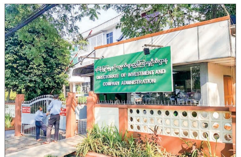
The office of the Directorate of Investment and Company Administration – DICA in Yangon.
