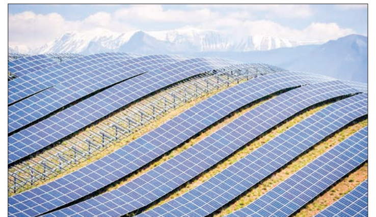
A general view shows the photovoltaic solar panels at the power plant in La Colle des Mees, Alpes de Haute Provence, southeastern France. PHOTO: GERARD JULIEN / AFP / FILE
