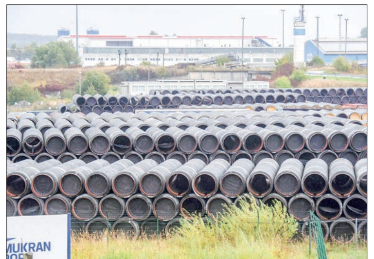
Unused pipes for the Nord Stream 2 Baltic gas pipeline stored on the site of the Port of Mukran in Lubmin, Germany. PHOTO: AFP
