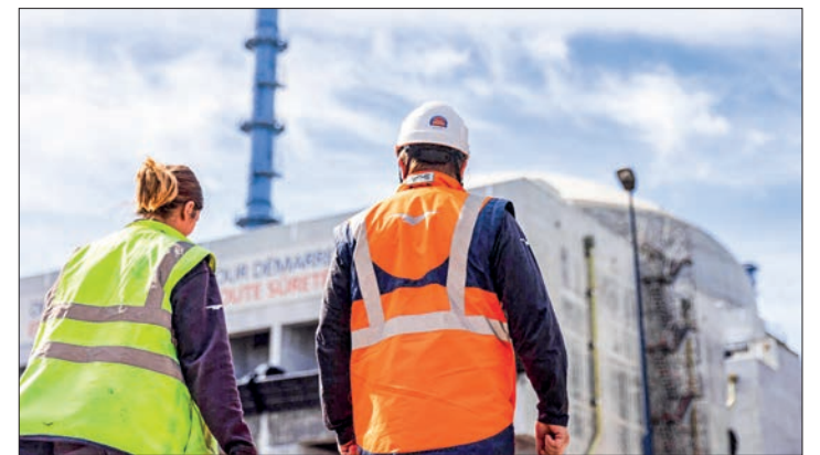
Workers walk past a reactor building at the third-generation European Pressurized Reactor project (EPR) nuclear reactor in Flamanville, Normandy, France on 14 June 2022. PHOTO: SAMEER AL-DOUMY /AFP
