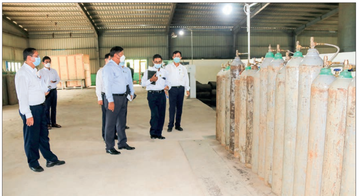
MoTC Union Minister Admiral Tin Aung San inspects the liquid oxygen plant in Dagon Myothit (Seikkan) Township.
