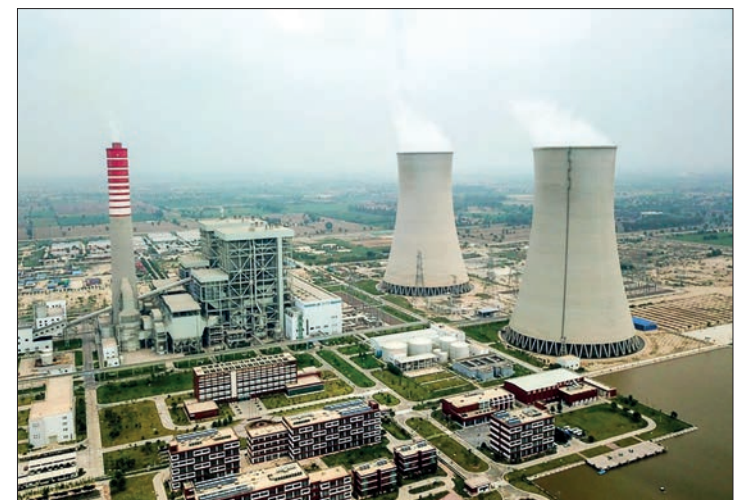
The aerial photo taken on 6 August 2019 shows the Sahiwal Coal Power plant in Sahiwal, Punjab Province, Pakistan. PHOTO: XINHUA/AHMAD KAMAL
