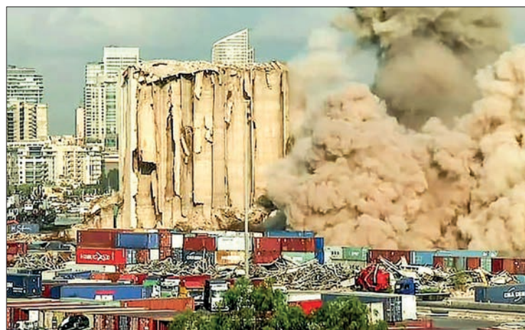
This grab from AFPTV footage shows a massive plume of smoke rising over Beirut port after the collapse of eight more grain silos damaged in a devastating 2020 explosion. PHOTO: AFP
