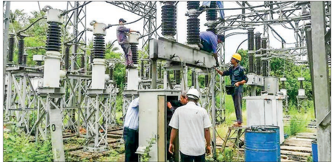
Workers repair electric transformers. PHOTO: YESC
