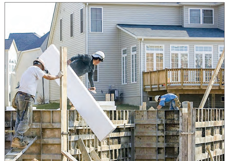
The continued slowing of housing starts is consistent with the expected impact of the monetary tightening on the slowing of economic activity. Construction workers place concrete forms into place for the base of a new single family home under construction in Centerville, Virginia. PHOTO: AFP / PAUL J. RICHARDS
