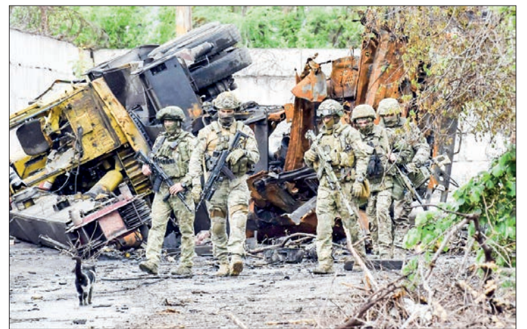
Russian servicemen patrol the destroyed part of the Ilyich Iron and Steel Works in Ukraine's port city of Mariupol on 18 May 2022, amid the ongoing Russian military action in Ukraine. PHOTO:AFP
