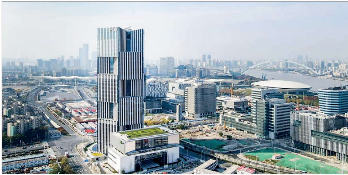
Aerial photo taken on 17 December 2020 shows the headquarters building of BRICS New Development Bank (NDB) in east China's Shanghai. PHOTO: XINHUA/FANG ZHE
