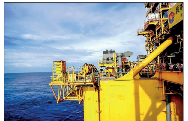
Photo taken on 8 June 2021 shows a partial view of the Deep Sea No. 1 oil production and storage facility located at Lingshui 17-2 gas field some 150 km off the island province of Hainan. PHOTO: XINHUA/ZHANG JIANSONG
