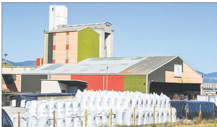
This photograph taken on 7 August 2020, shows a general view of "Engrais Sud Vienne," a company where fertilizer and ammonium nitrate are believed to be stored, at Salaise-sur-Sanne, France.
