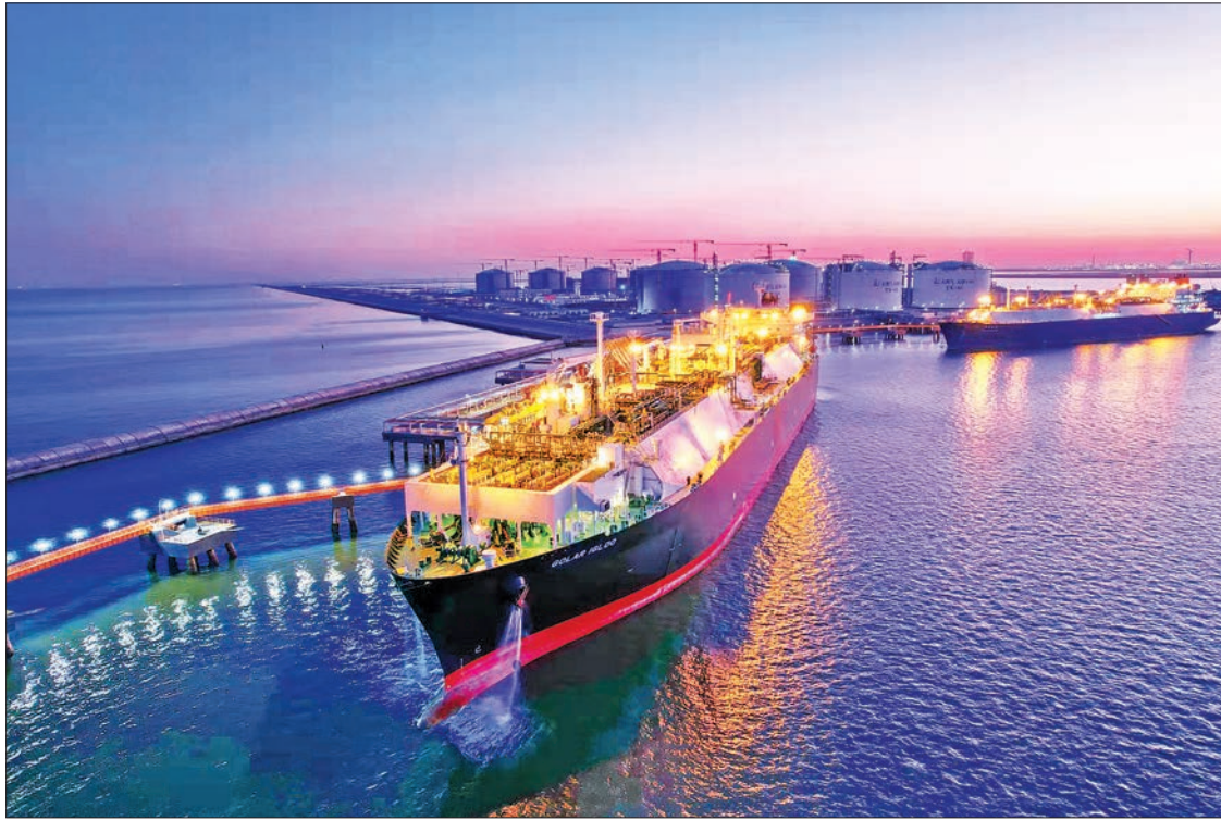
The liquefied natural gas (LNG) terminal of Sinopec Tianranqi Company in north China's Tianjin municipality, the first LNG terminal with two berths in China, receives two batches of LNG at the same time, 26 Feb 2022. (Photo by Hu Qingming/People's Daily Online)
