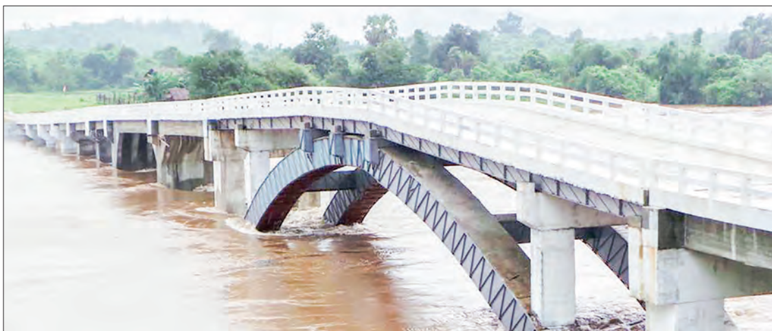
A bridge is lying across a creek for smooth transportation.
