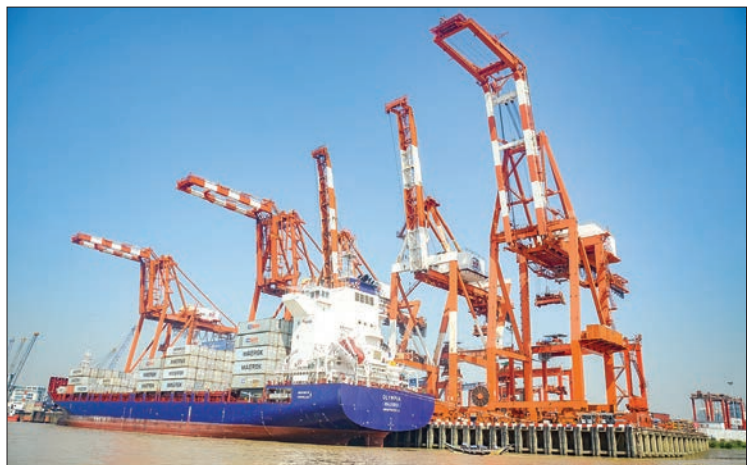
The country currently has nine ports involved in sea trade. Yangon Port is the main gateway for Myanmar’s maritime trade and includes the Yangon inner terminals and the outer Thilawa Port.
