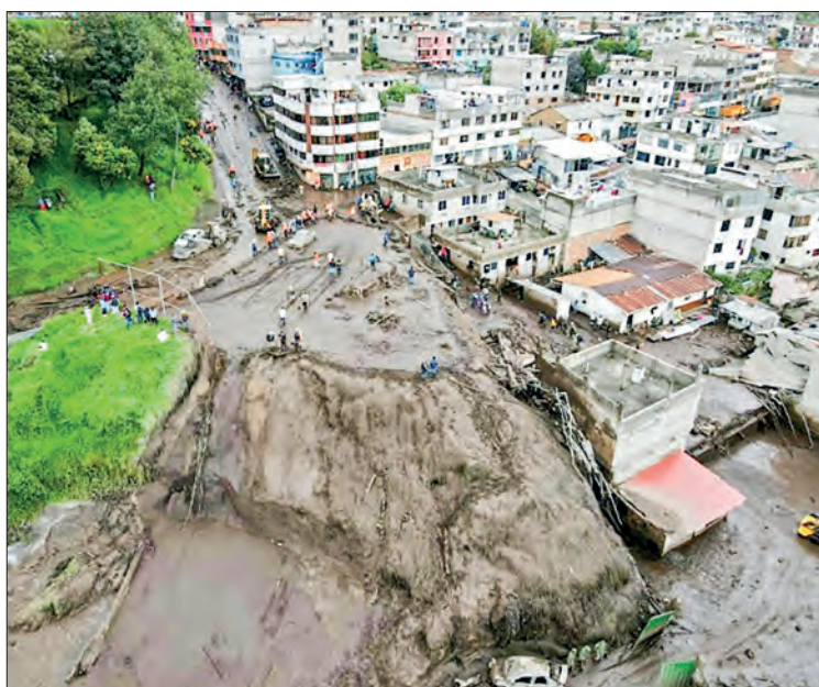
An areal view of the damage in the neighbourhood of La Gasca.
