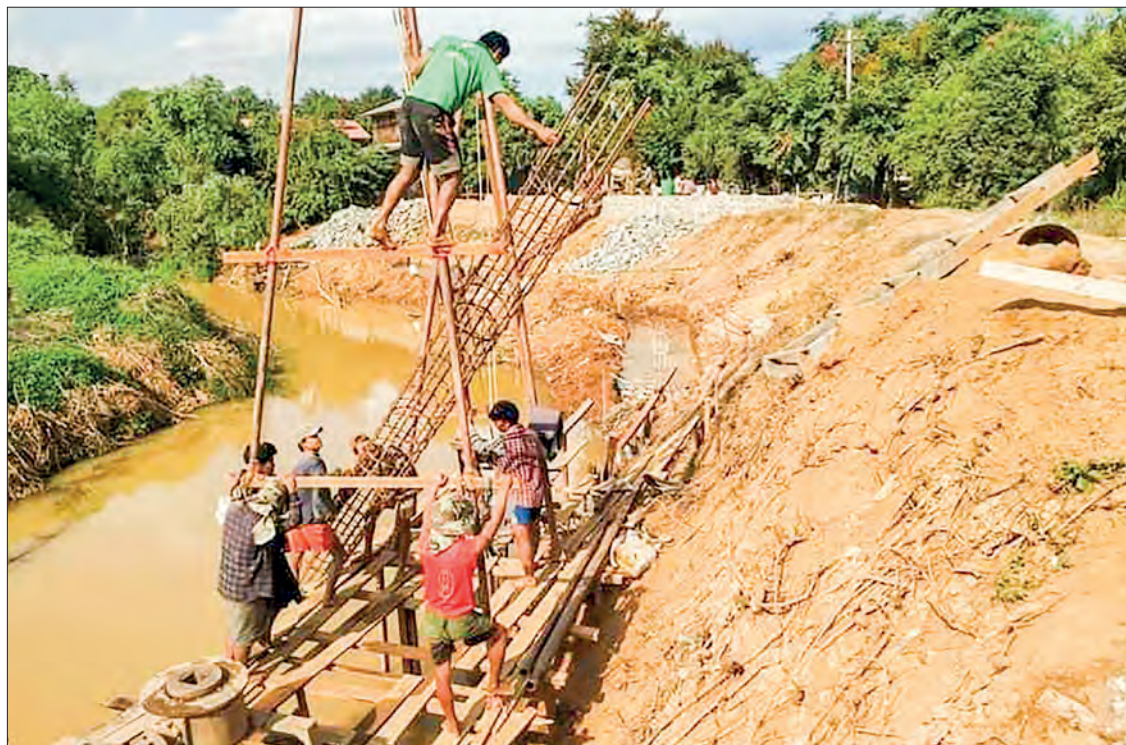
The Daungmyu Creek landslide protection project is underway.
