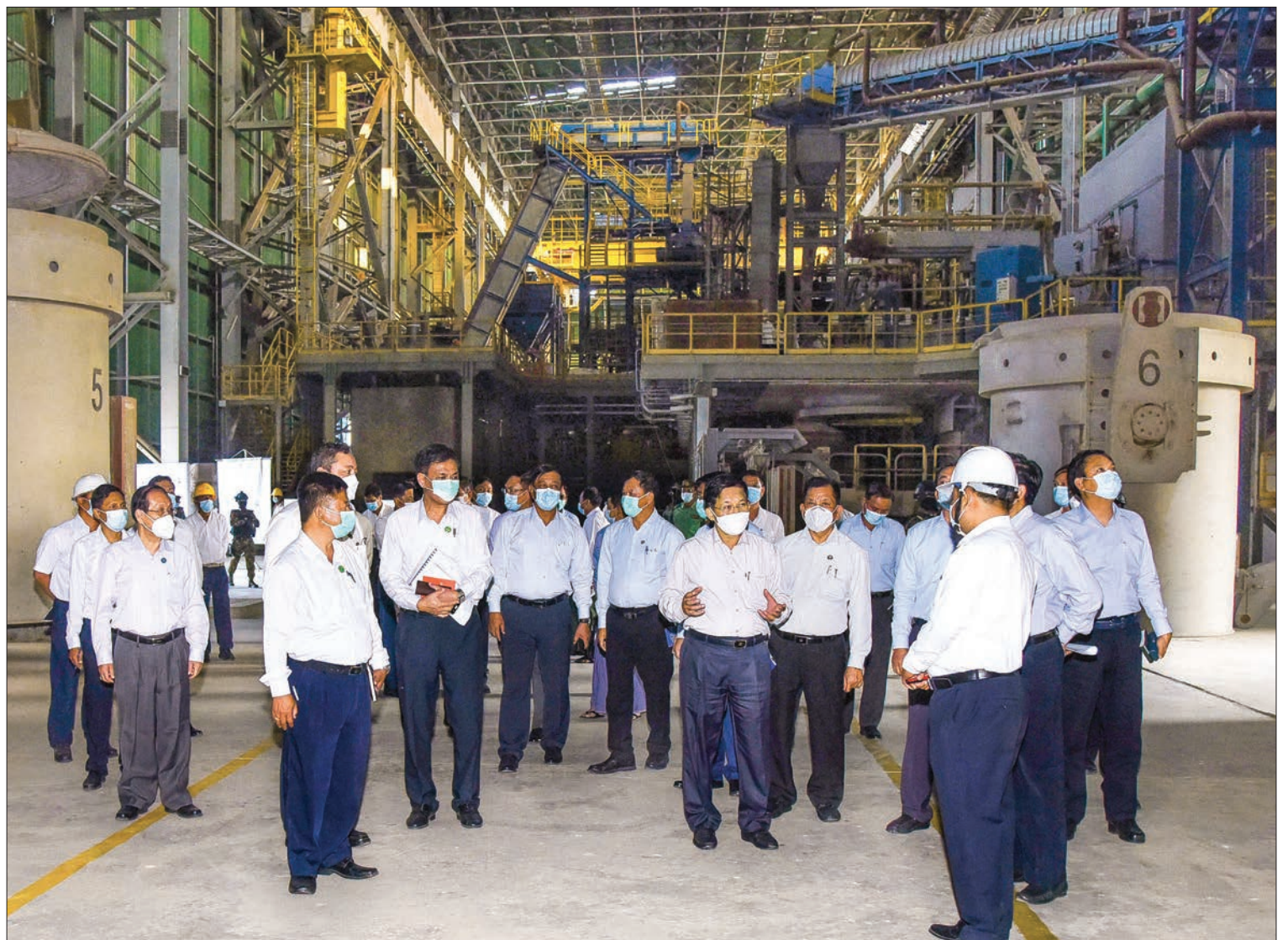
State Administration Council Chairman Prime Minister Senior General Min Aung Hlaing inspects No 1 Steel Mill (Myingyan) of the Ministry of Industry in Myingyan Township, Mandalay Region on 24 January 2022.
