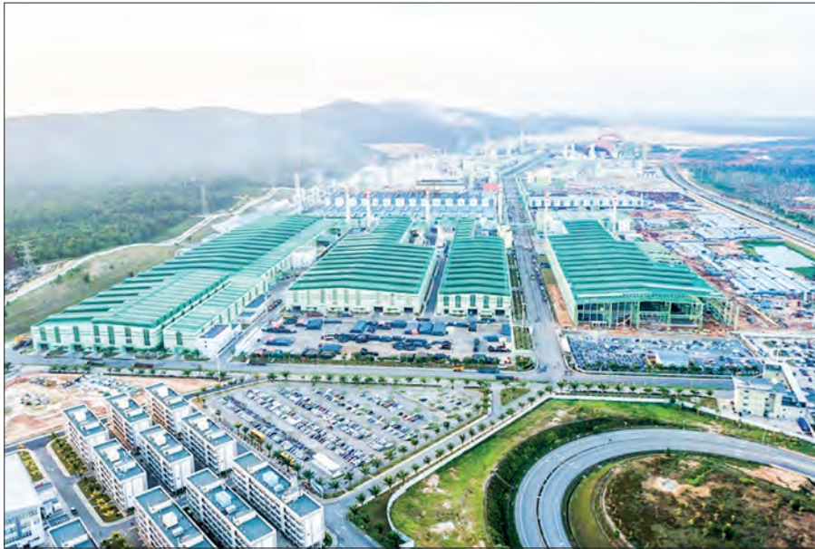
Aerial photo taken on 15 April 2019 shows the Alliance Steel at the Malaysia-China Kuantan Industrial Park in Pahang, Malaysia. PHOTO: XINHUA/ZHU WEI
