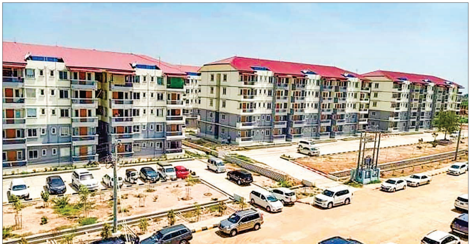
One of the public rental housing projects in progress. PHOTO: MOC
