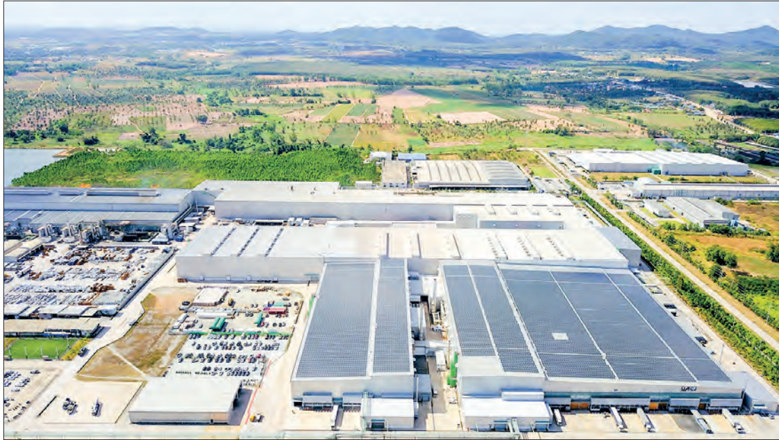
Aerial photo taken on 29 December 2021 shows the Thai-Chinese Rayong Industrial Zone. PHOTO: XINHUA/WANG TENG
