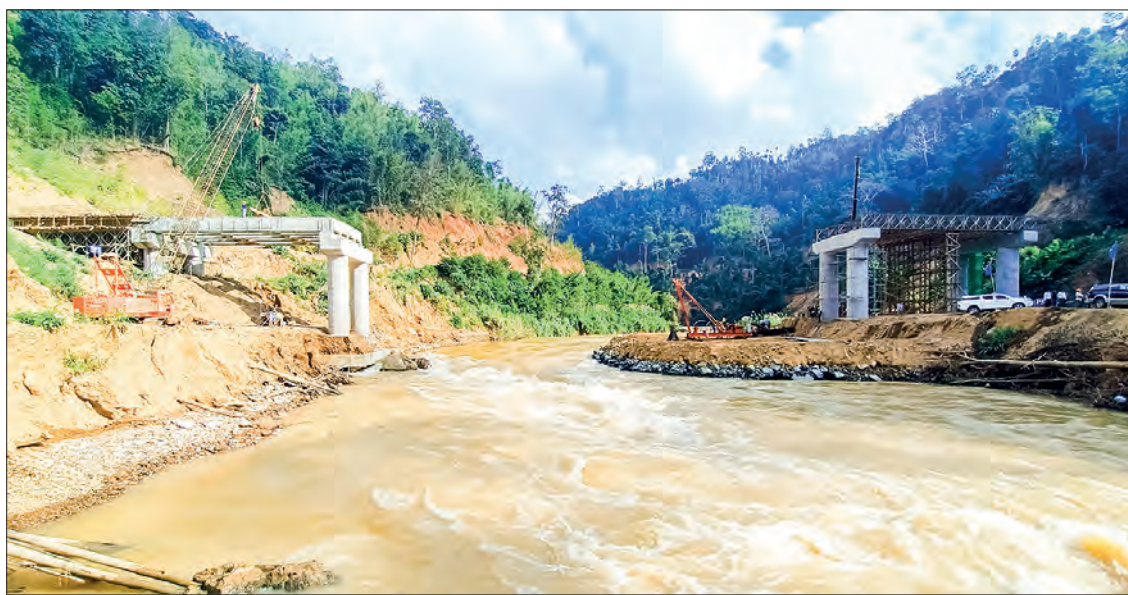
The construction site of the Middle Paunglaung Bridge.
