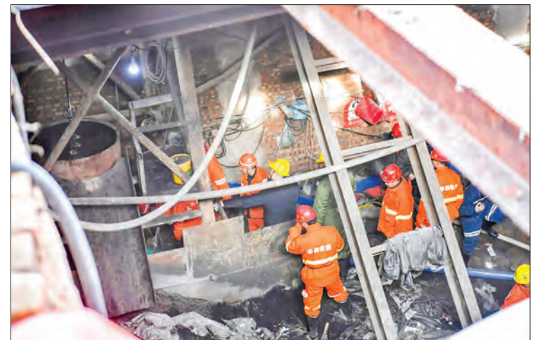
In this photo released by China’s Xinhua News Agency, rescuers work at a coal mine at Duxigou Village of Xixinzhuang Township in Xiaoyi City in northern China’s Shanxi Province, Thursday, 16 December 2021. More than 20 people were trapped after a coal mine was flooded in the city of Xiaoyi, north China’s Shanxi province, as a result of illegal mining, local authorities said Thursday. PHOTO: CAO YANG/XINHUA
