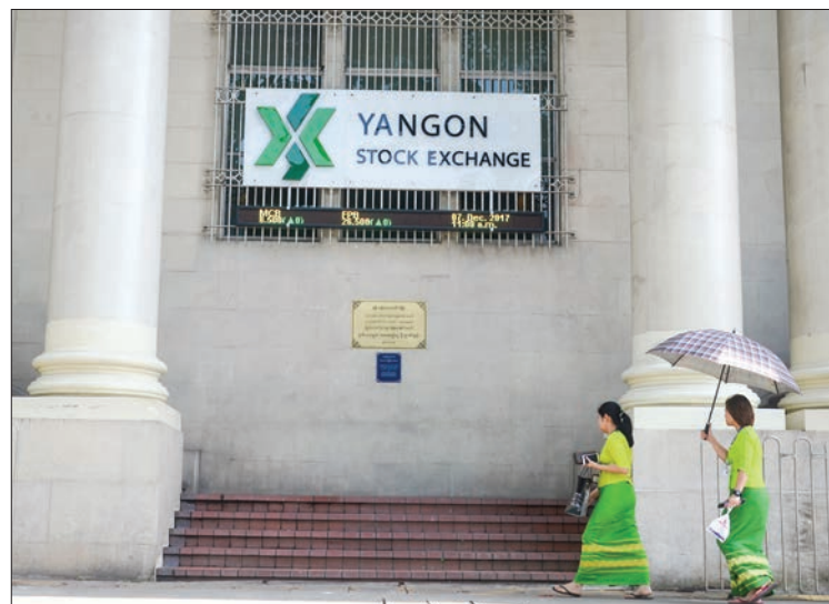
Photo shows building of Yangon Stock Exchange in Yangon Region.
