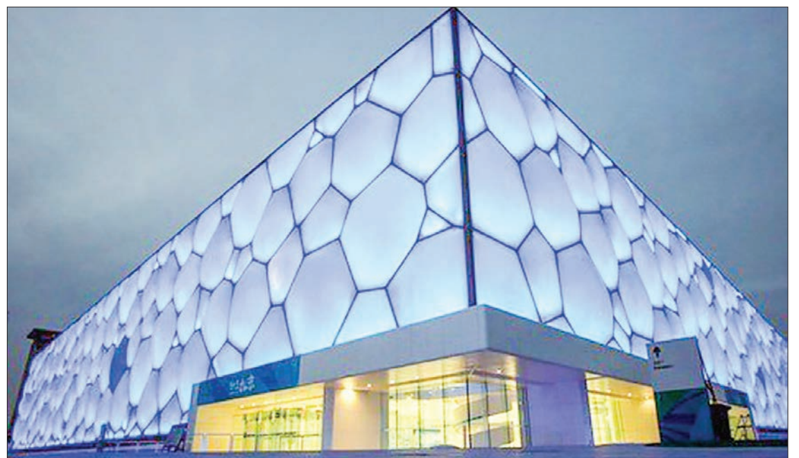
The 'Ice Cube' venue will operate at 20 per cent capacity during the Beijing Winter Olympics over Covid fears, its manager told Chinese state media. The exterior view of the National Aquatics Centre PHOTO: XINHUA / FILE
