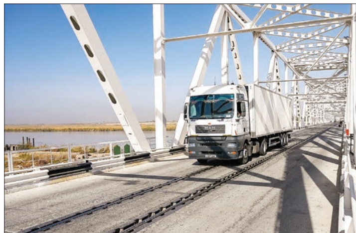
This picture taken on 27 October 2021 shows a truck arriving from Uzbekistan at the Afghanistan-Uzbekistan Friendship Bridge in Hairatan, about 82 kms north of Mazar-i-Sharif. PHOTO: AFP
