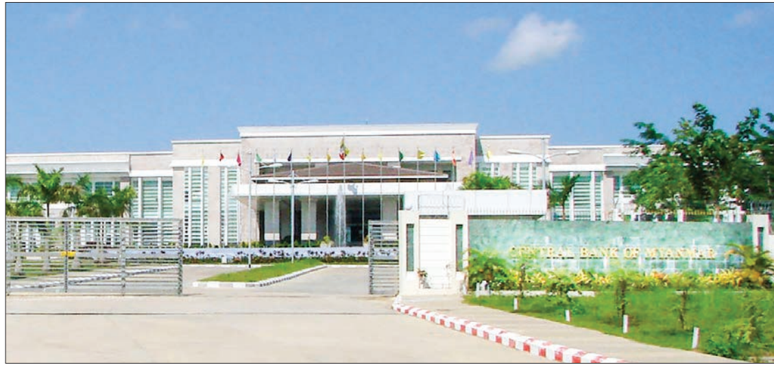
Photo depicts building of Central Bank of Myanmar.
