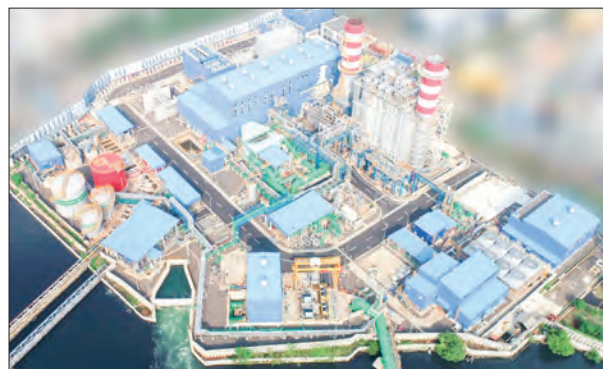
Photo shows the Muara Karang power plant on Indonesia's Java island, where Japan's Mitsubishi Heavy Industries Ltd. provided a 500-megawatt natural gas-fired gas turbine combined power generation system. PHOTO: KYODO NEWS
