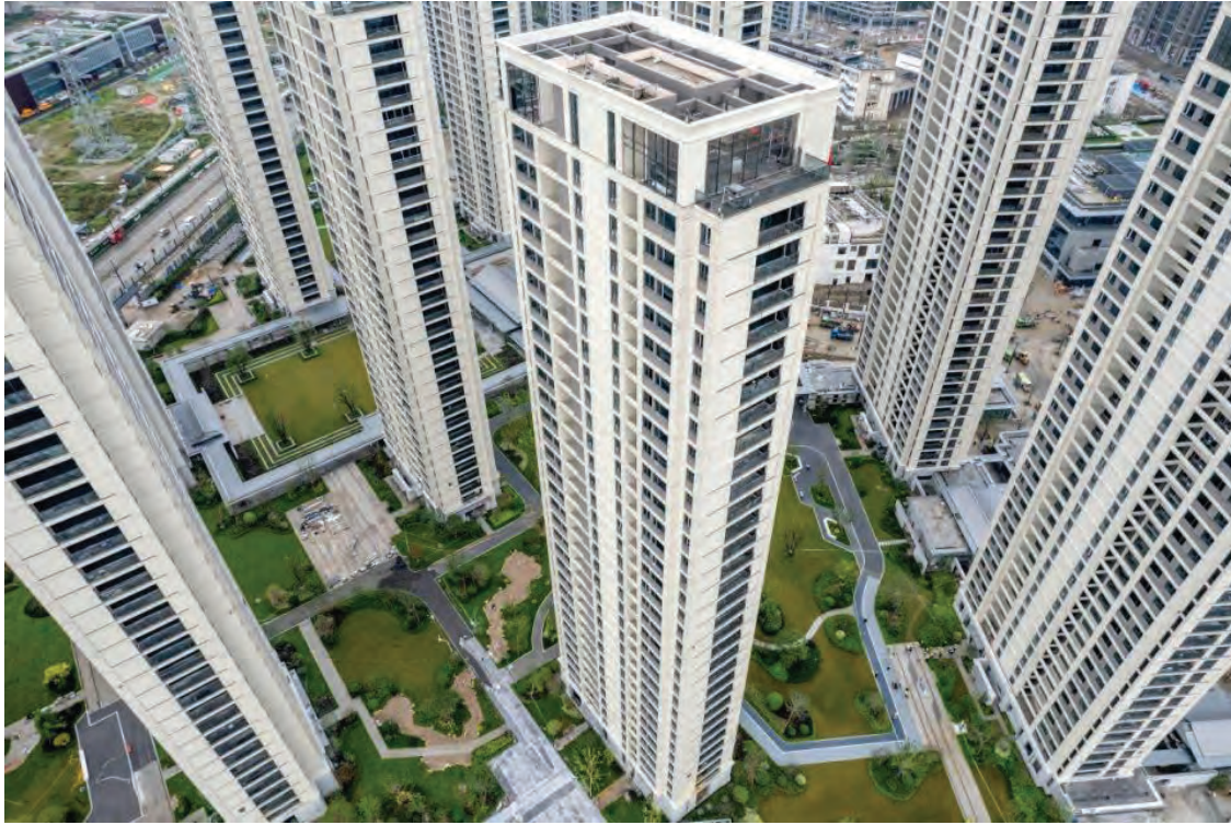
The Hangzhou Asian Games village housing under construction in preparation for the 2022 Asian Games in Hangzhou, China. Property and construction are pillars of the Chinese economy, underpinning other important sectors such as commodities and furnishings. PHOTO: DAN SANDOVAL / PUBLICITY DEPARTMENT OF HANGZHOU/AFP
